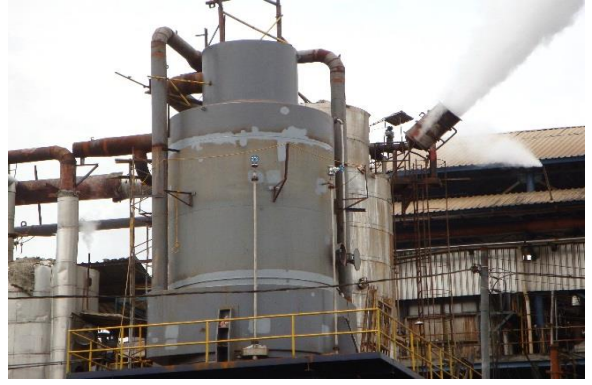
Ilustración 65: Equipo montado antes de operación. A photograph showing the same industrial tank fully assembled and operational. A large plume of white steam or smoke is being emitted from a pipe on the right side of the tank. The tank is surrounded by a complex network of pipes and structural elements.
